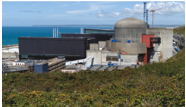
Figure E.4: External containment of an operating PWR plant
