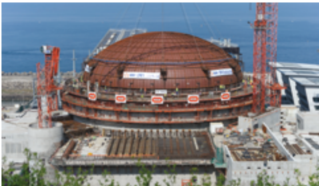
Figure E.3: Flamanville PWR plant under construction
